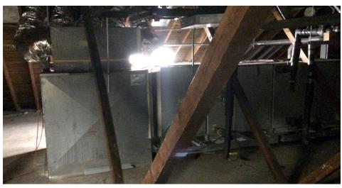
heavy material gauges allow for longer equipment life as compared to cataloged constructed units commonly found in the market place. The AHUs installed comprised of filters, coils, FANWALL Technology, variable frequency drives, airflow monitoring,
